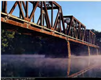
Former Eastern RR Bridge, later acquired by Boston and Maine RR
