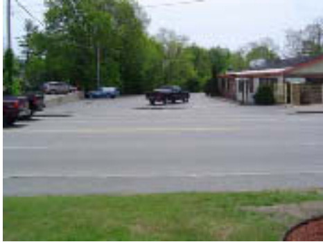
Excessively Wide Driveway at The China House Restaurant
