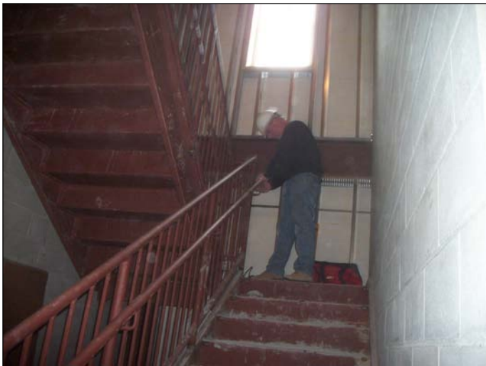
Photo 19 (1453) : Shows Davis Erectors Co. crew repairing handrails in the stairway.
