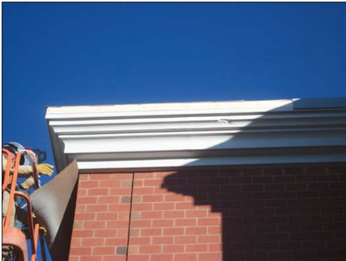
Photo 13 (1427): Shows SMR Roofing Co. crew installing flashing on the roof parapet.
