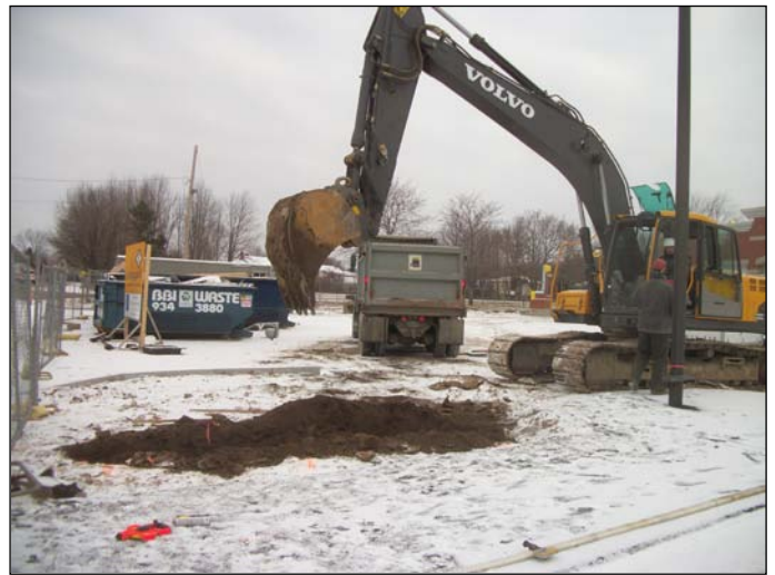
Photo 18 (1449): Shows Peters Construction Co. crew excavating for the sign base.
