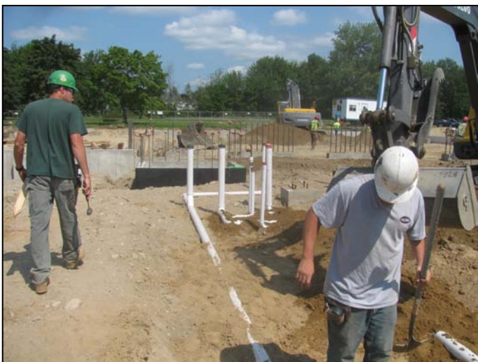
Photo 3 (4569) Shows Titon Mechanical Co. crew installing underslab sanitary piping.
