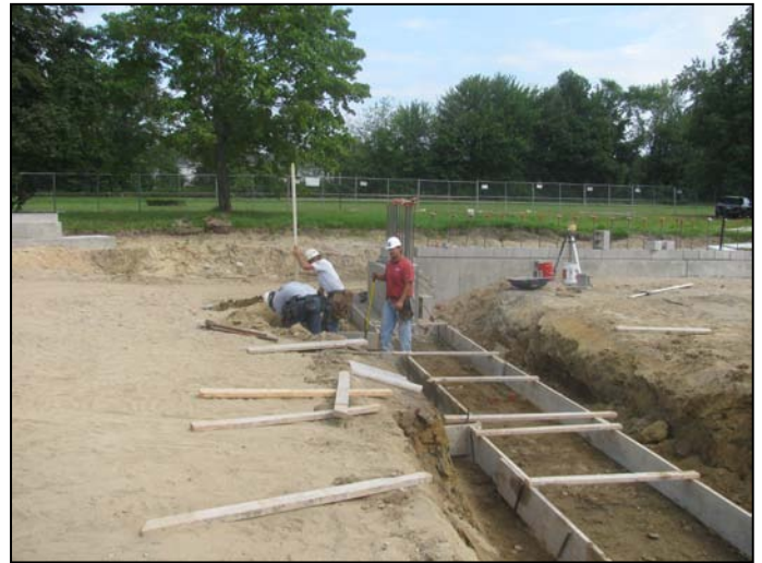
Photo 6 (4589) : Shows Lajoie Bros. Construction Co. crew forming west wall foundation footing.
