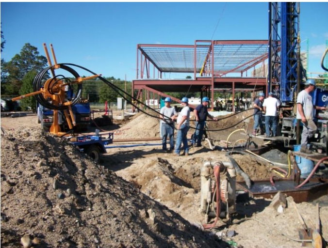
Photo 11 (0043): Shows Goodwin Well Drilling Co. crew installing geothermal piping in well No. 8.
