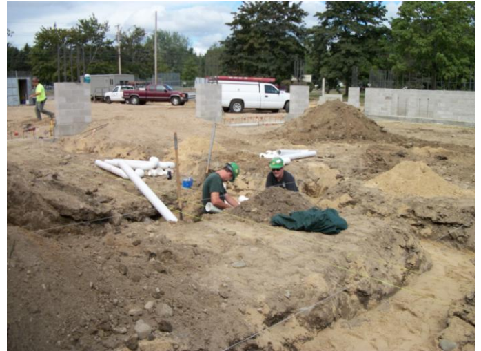
Photo 2 (030): Shows Titan Mechanical Co. crew installing sanitary drain piping below the floor slab in the Apparatus Bay area.
