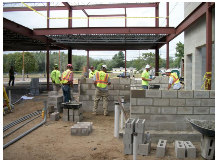
Photo 4 (031): Shows Nate Libby Masonry Co. crew installing concrete masonry units on stairwell No. 1.
