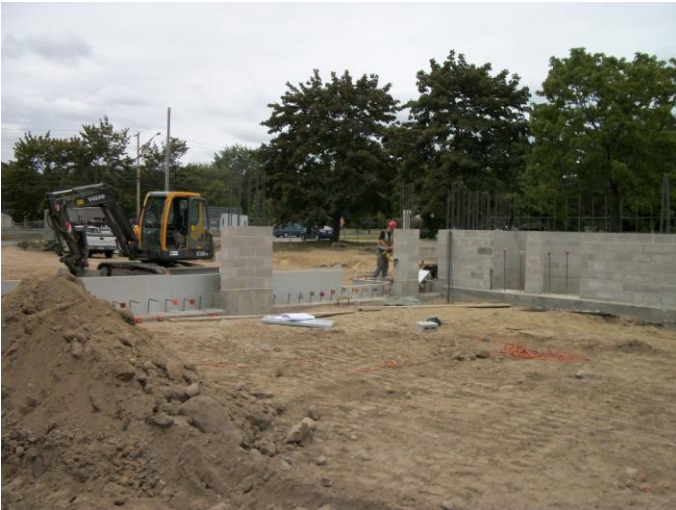
Photo 1 (039): Shows Peters Construction Co. crew installing exterior insulation at the foundation wall of the Apparatus Bay west wall.
