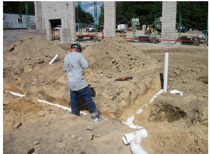
Photo 12 (0066): Shows Titan Mechanical Co. crew installing sanitary drain piping in the Apparatus Bay, excavations performed by Peters Construction Co. crew.
