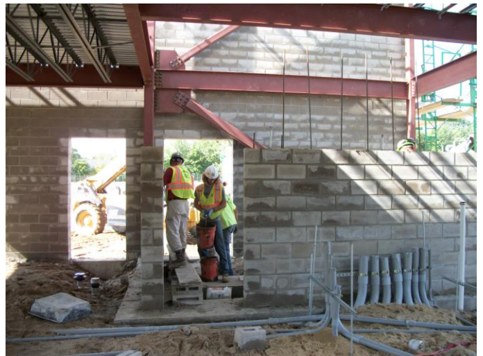
Photo 8 (0051) : Shows Nate Libby Masonry Co. crew installing concrete blocks in stairwells No. 1 and 2.
