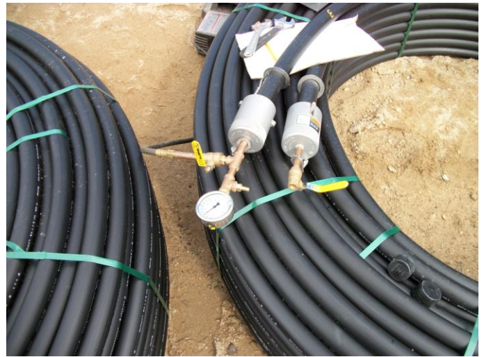
Photo 6 (027) : Shows Gillespie testing the geothermal well piping.
