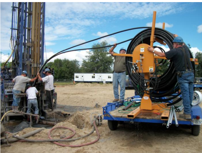
Photo 3 (038): Shows Goodwin Well Drilling Co. crew installing the piping in geothermal well No. 10.
