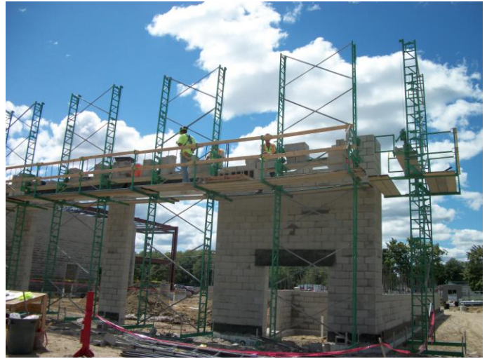
Photo 14 (0059) : Shows Nate Libby Masonry Co. crew installing masonry blocks on east wall of the Apparatus Bay.
