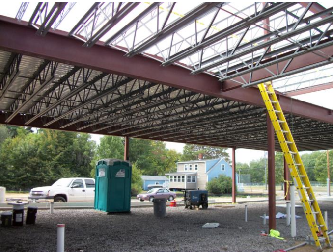
Photo 5 (033) : Shows Davis Erectors Co. crew installing decking on second floor elevation in the Administration area.
