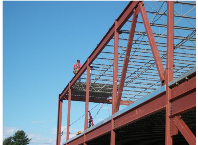
Photo 10 (0041): Shows Davis Erectors Co. crew working on roof decking.
