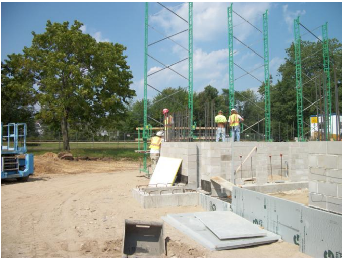
Photo 15 (0138): Shows Nate Libby Masonry Co. crew installing concrete blocks on north wall of the Apparatus Bay.
