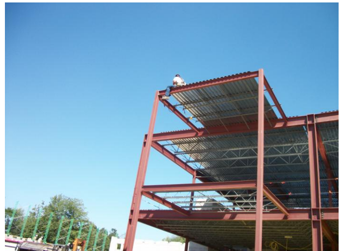
Photo 22 (0159): Shows Davis Erectors Co. crew welding roof decking.
