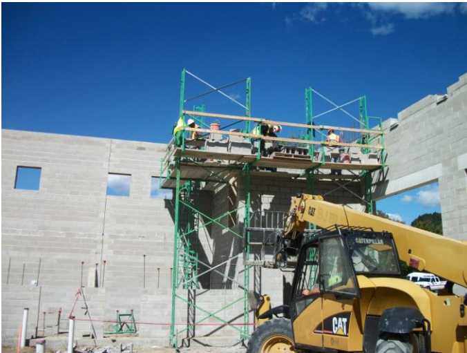
Photo 3 (0318): Shows Nate Libby Masonry Construction Co. crew installing concrete blocks in training tower walls.
