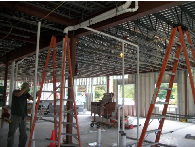
Photo 15 (0385): Shows Titan Mechanical Co. crew installing plumbing piping
