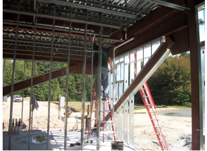
Photo 2 (0320): Shows B.H. Milliken Electrical Co. crew installing conduits in the Administration Area.
