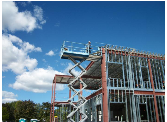
Photo 4 (0326): Shows Dirago Drywall Co. crew installing framing in parapet walls in Administration Area.
