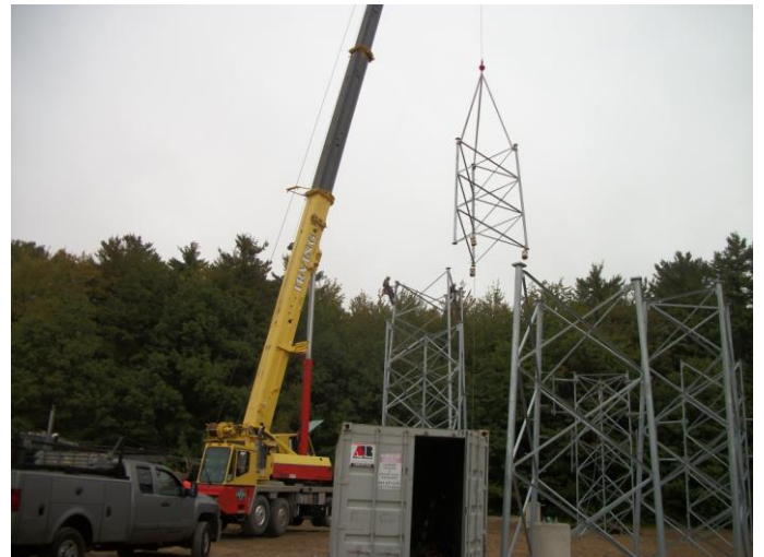
Photo 4 (0409): Shows Green Mountain Communication Co. crew erecting the communication tower.
