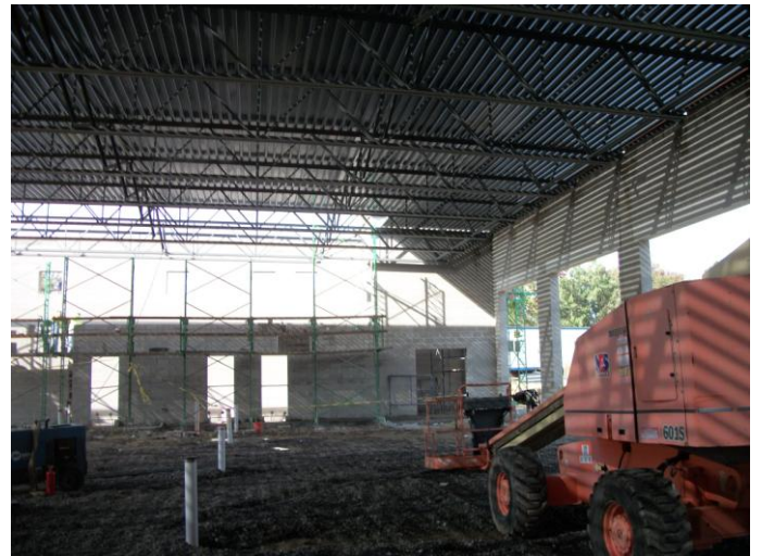
Photo 12 (0463) : Shows Davis Erectors installing roof decking on the Apparatus Bay area.
