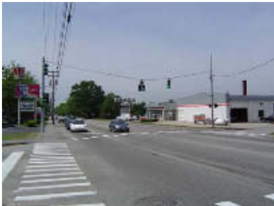
Signalized Intersection at Hutchins Avenue
