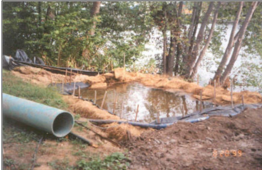
***A temporary sedimentation basin, silt fence and hay bales were utilized at the area of the trunk outfall to protect the Saco River from suspended solids and erosion (Spring Street Trunk Storm Drain Project).***
